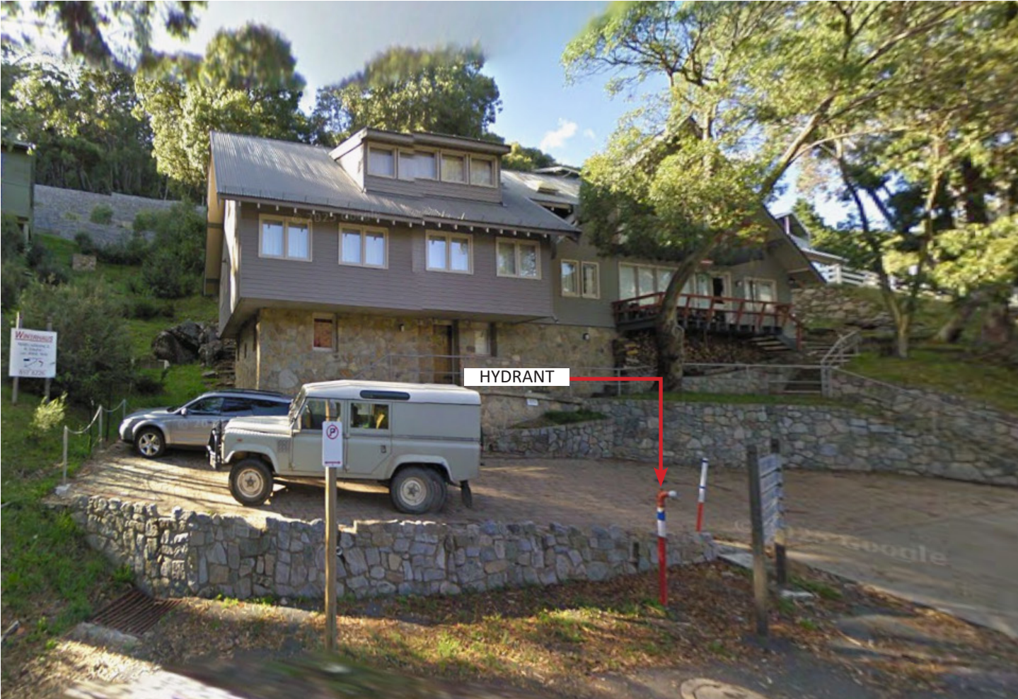
05 : Hydrant located at the property entrance.
